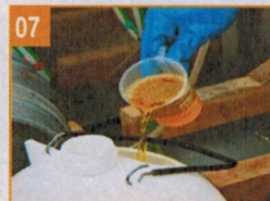
07 Fill vessel with Pipeline Gold Professional and top up with water
