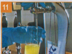
11 Draw cleaning fluid through tap until visible
