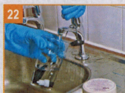
22 Rinse tap fittings & re-fit
